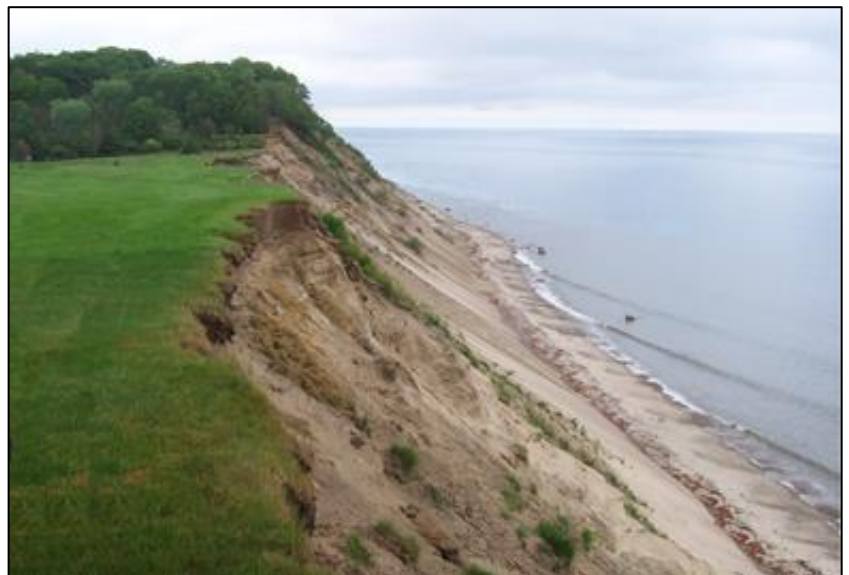
Extensive irrigated lawns that slope seaward have exacerbated the erosion of this coastal bank. (Photo: CZM)
