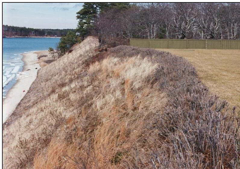
This lawn was regraded to slope inland, and a buffer of native shrubs was planted along the top of the bank to stabilize the area and direct runoff away from the bank. These measures reduced runoff flowing over the bank so that a bioengineering project with natural fiber blankets, coir rolls, and vegetation could be successfully installed. (Photo: CZM)
