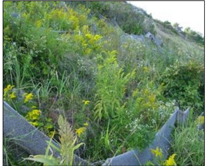
Lightweight, natural-fiber, erosion-control fabric was installed on this bank to protect the plants from wind until the roots could get established. Boards were placed on top of wooden stakes to provide access during construction, which minimized impacts to the bank from foot traffic. The photo on the right was taken one year after planting. (Photos: New England Environmental, Inc.)
