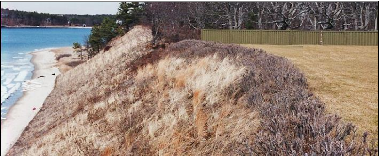
Shrubs were planted at the top of this bank to slow runoff. On the bank face, natural fiber blankets were installed to hold soils in place until the erosion-control vegetation could get established. (Photo: CZM)
